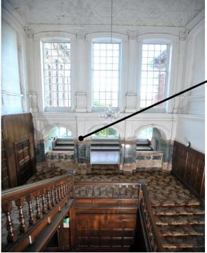
A panel of Marble installed 1936 – 40 has been smashed whilst trying to be removed
