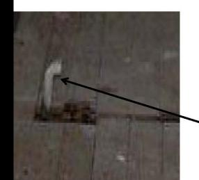
WHEN DERBYSHIRE INVESTMENTS REMOVED THE EN-SUITE BATHROOMS AND TOILETS THEY REMOVED ALL THE PARTITION WALLS LEAVING GAPS IN THE FLOORS BUT MORE IMPORTANTLY THEY DID NOT CAP OFF THE WATER PIPES. INSTEAD THEY SIMPLY CRIMPED THE ENDS OF THE PIPES AS IS THE CASE WITH THE PIPES IN THIS ROOM ON THE WEST FRONT OF THE HALL ON THE FIRST FLOOR AS A RESULT THERE IS A STRONG POSSIBILITY THAT IF THE MAINS ARE TURNED BACK ON FROM THE STOP TAP BY THE CROSS ROADS. THE HALL WILL FLOOD
