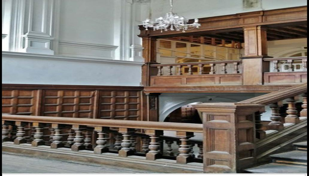
The Main Staircase. Showing the false ceiling installed by the Vinces to reduce heating cost and create a fire break. Nesfield's original ceiling is above this
