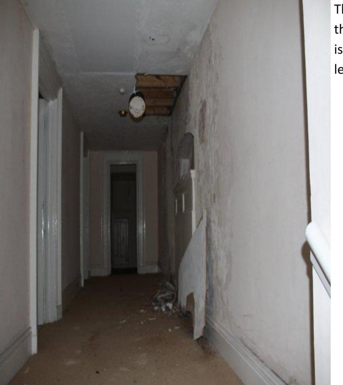
This is the Second Floor Landing on the East Front. The Collapsed Ceiling is a long standing problem due to a leak in the roof
