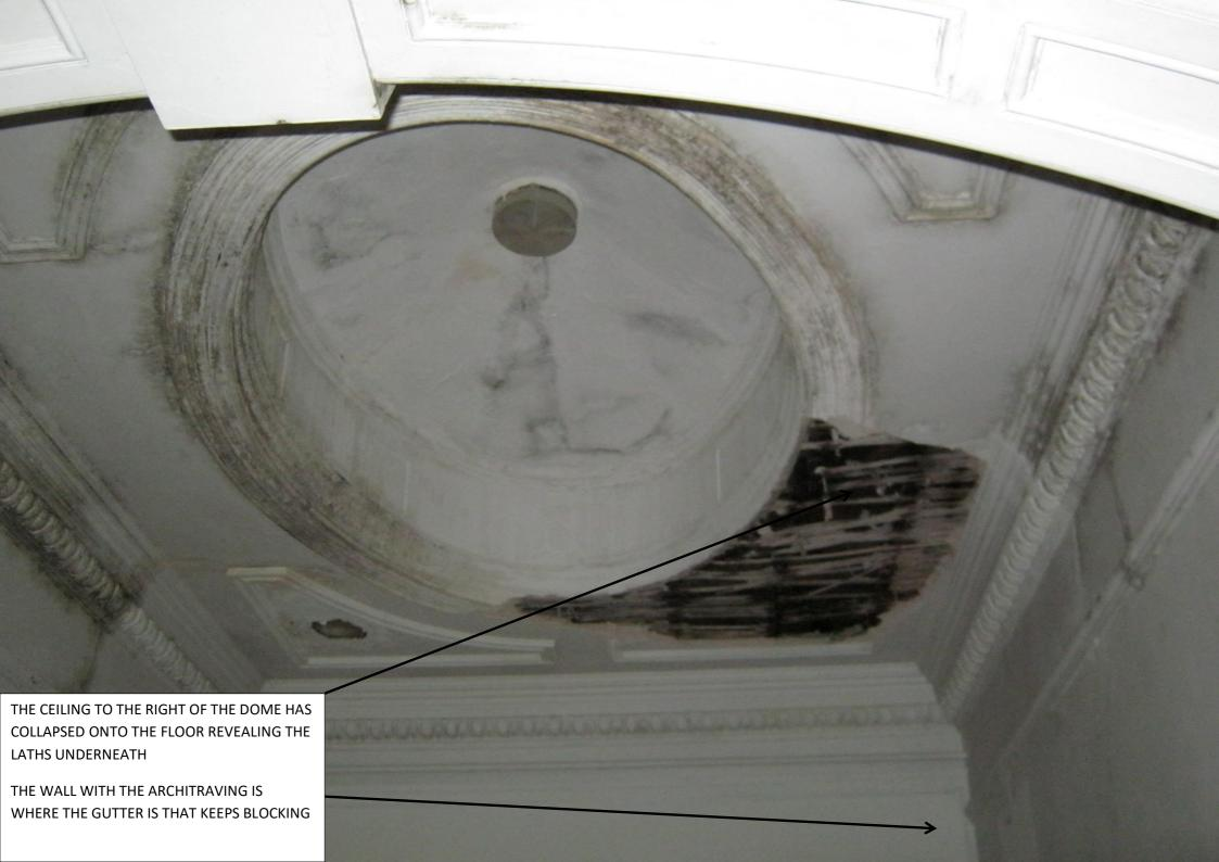
During the rebuilding of Kinmel Hall an error was made with the drainage that runs across the roof of the Ballroom adjoining the end wall of the SECOND FLOOR Corridor (as shown in the photo).
