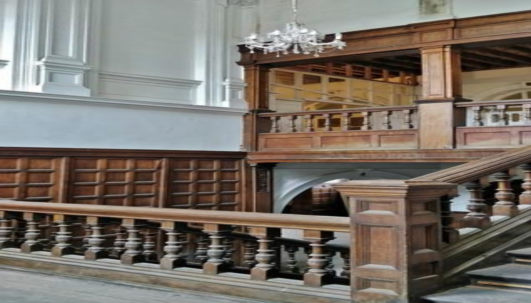
The Main Staircase. Showing the false ceiling installed by the Vincés to reduce heating cost and create a fire break. Nesfield's original ceiling is above this
