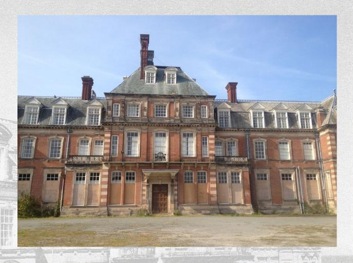
This was the workmen's interpretation to these instructions. To make matters worse the wooden panels have been screwed into the wooden window frames – without Listed Planning Consent.
